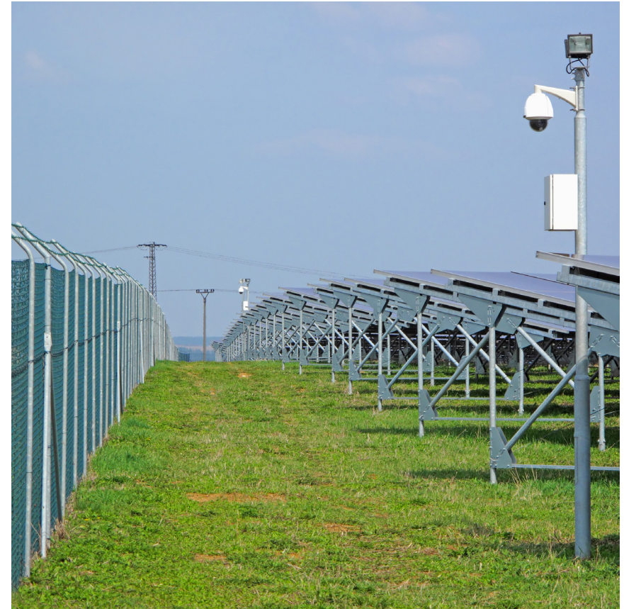
Multi-layered security at a solar park may include fence-mounted perimeter intrusion detection sensors, AI-powered analytics, and security lighting.
