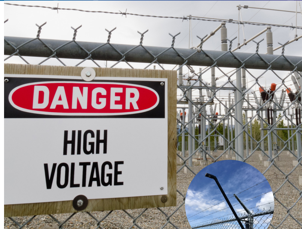
Senstar LM100 luminaire
