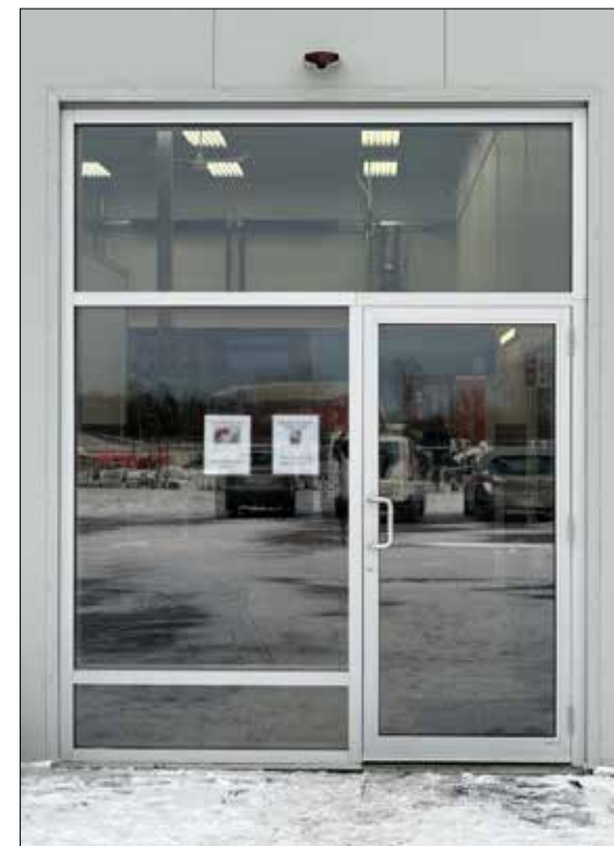
An example installation in which Senstar MultiSensor monitors a public entrance.
