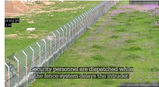
Surveillance footage of a FiberPatrol fiber optic perimeter intrusion system detecting an intrusion attempt and reporting the location to the Symphony VMS
