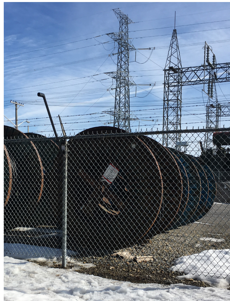
Senstar LM100 Intrusion Detection and Deterrence System protecting an electrical storage yard.
