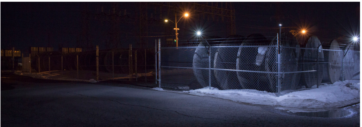
This example shows the difference between having Senstar LM100 on the fence (right) and not
