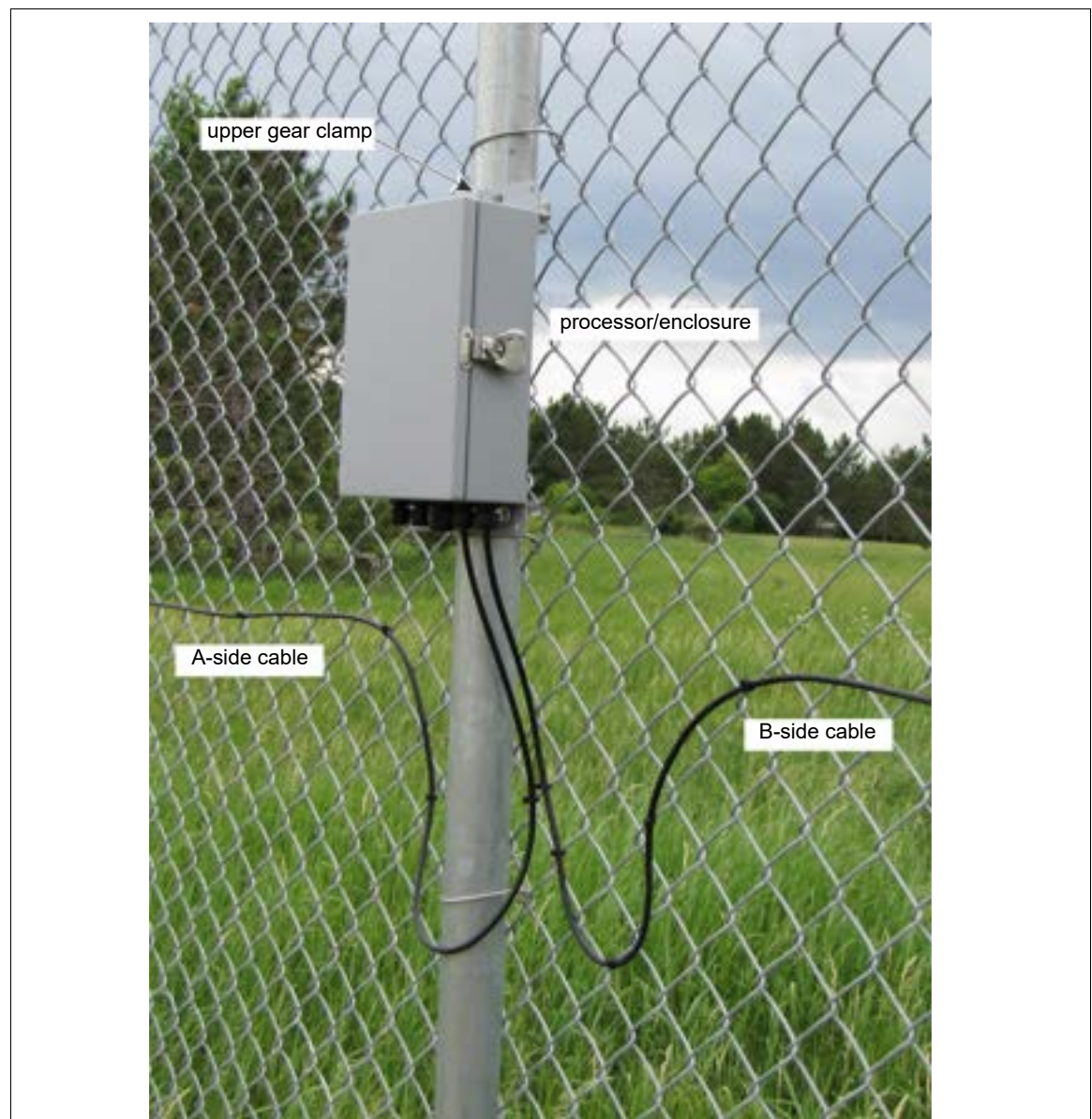
Figure 62: FlexZone single pass dual zone fence-mounted processor
