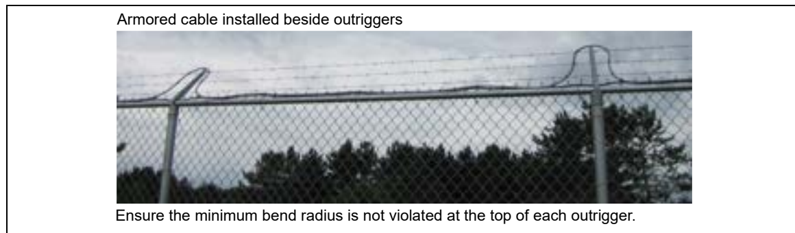
Figure 51: Armored cable installation on barbed wire
