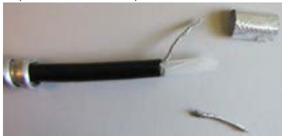
Figure 54: Armored cable preparation for splicing
