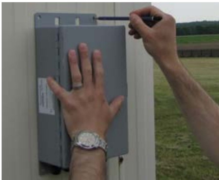
Figure 64: Surface-mounting the enclosure
