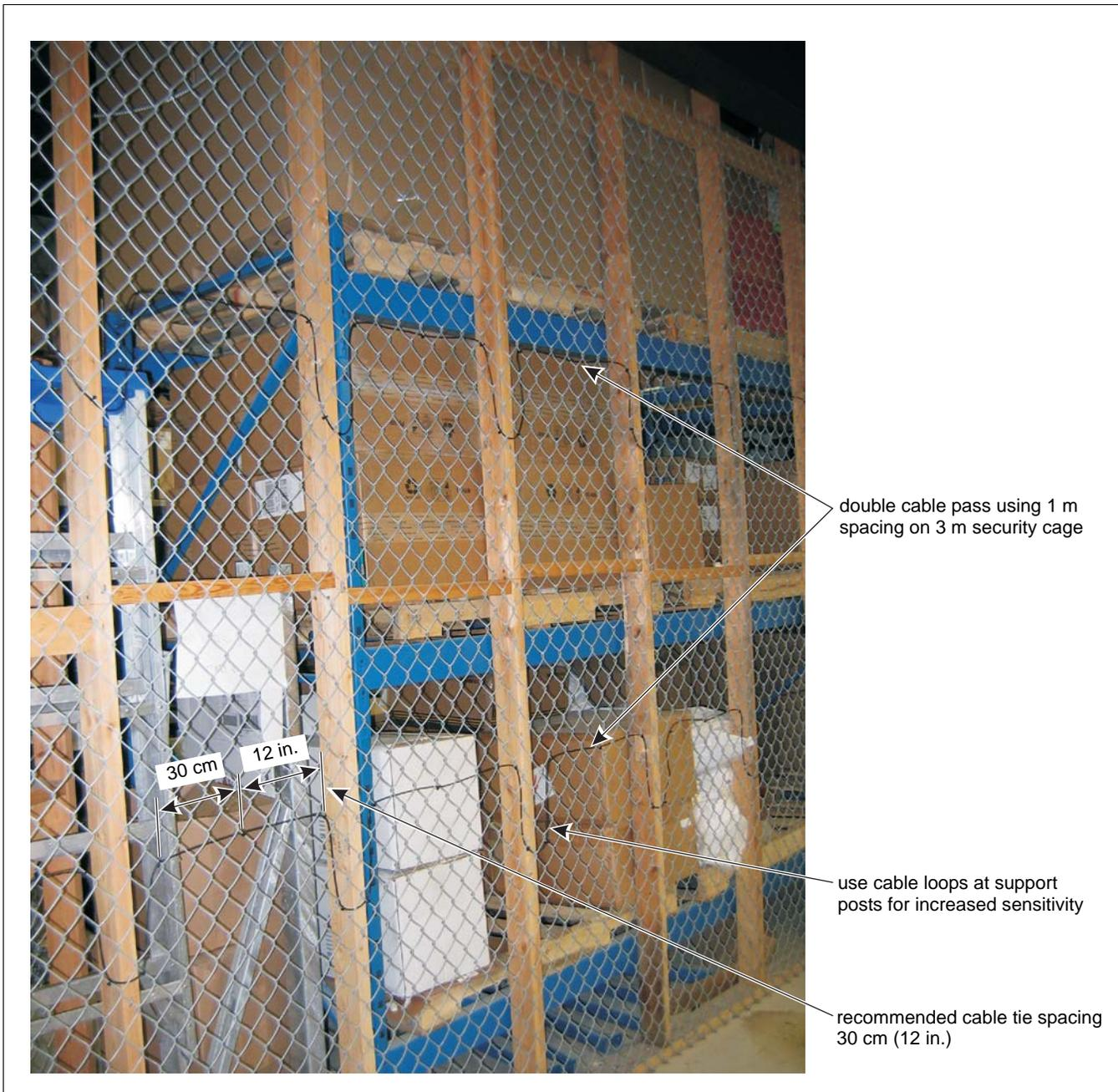
Figure 2: Double pass security cage installation
