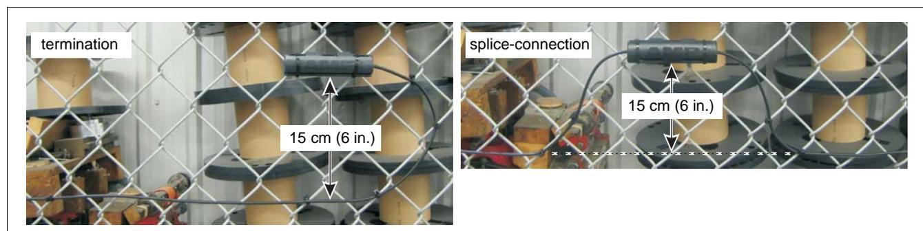
Figure 19: Creating drip loops for outdoor terminations/splice-connections
