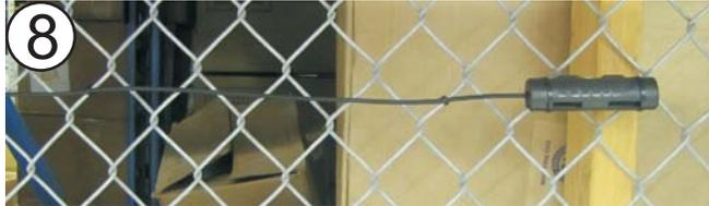
Figure 17: Terminating the sensor cable
