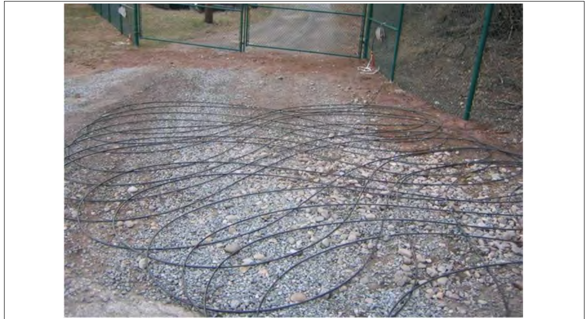
Figure 36 Laying cable in a figure-8 pattern
