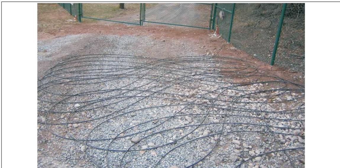
Figure 56 Laying cable in a figure-8 pattern
