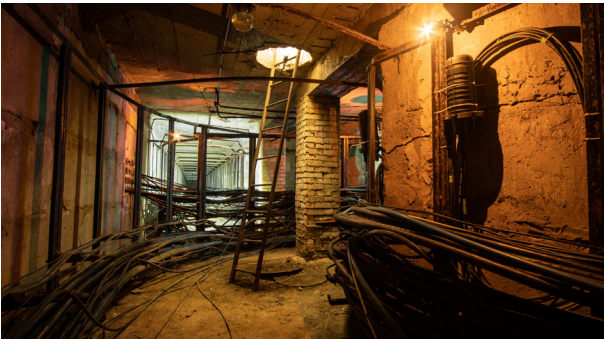
In urban areas, communication lines may be installed in legacy service tunnels and be relatively unprotected from nearby maintenance or construction activities.
