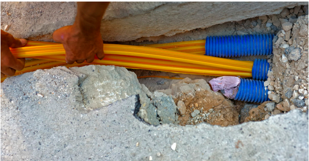
FiberPatrol for data conduit detects and locates any disturbance to the communications conduit, including nearby machine and human digging.
