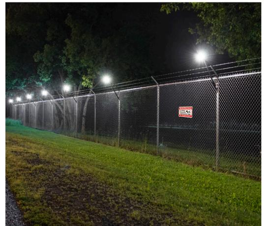
The Senstar LM100 Perimeter Intrusion Detection and Intelligent Lighting System uses an encrypted self-healing wireless mesh network for communication between luminaires. This eliminates the need to run communications wiring along the fence. The mesh network also maintains communications if several of the fixtures are physically damaged or have their power supply cut off.
