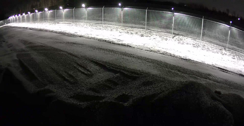
This capture from a surveillance camera demonstrates the light falloff of the Senstar LM100. Targeted illumination along the fenceline ensures the perimeter is well lit and free of hotspots while avoiding light encroachment onto nearby areas.
