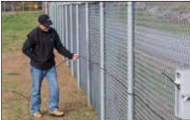
4. Connect power, communications wiring, and sensor cable to the processor. Removable connectors make it easy to attach the wires.
