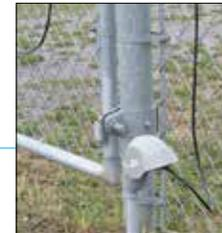
The FlexZone sensor cable can be installed directly on single and double swinging gates. To get to the other side, the cable is routed underneath the gate in buried conduit.
