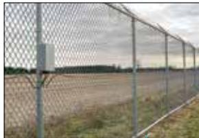
The FlexZone sensor detects any attempt to cut, climb, or lift the fence fabric. When properly installed, the sensor cables are guaranteed to work in all weather conditions and have a minimum service-life of 10 years†.
