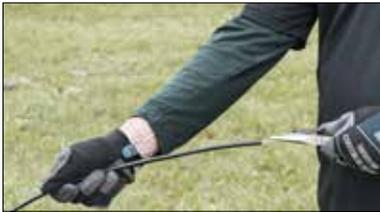
3. Attach the sensor cable along the fence (typically mid-way up) using UV-rated tie wraps. Extra cable should be placed on the fence near corners and other reinforced areas. At gates, the cable is tunneled in conduit underneath to the other side.
