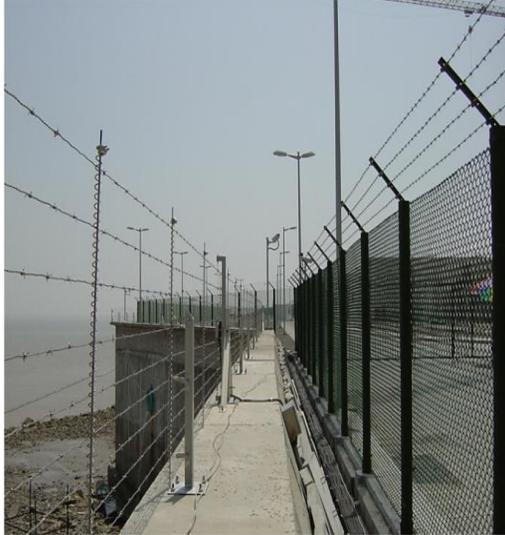
*A multi-layer power plant security scheme with outer taut wire and inner microphonic fence-mounted sensors*
