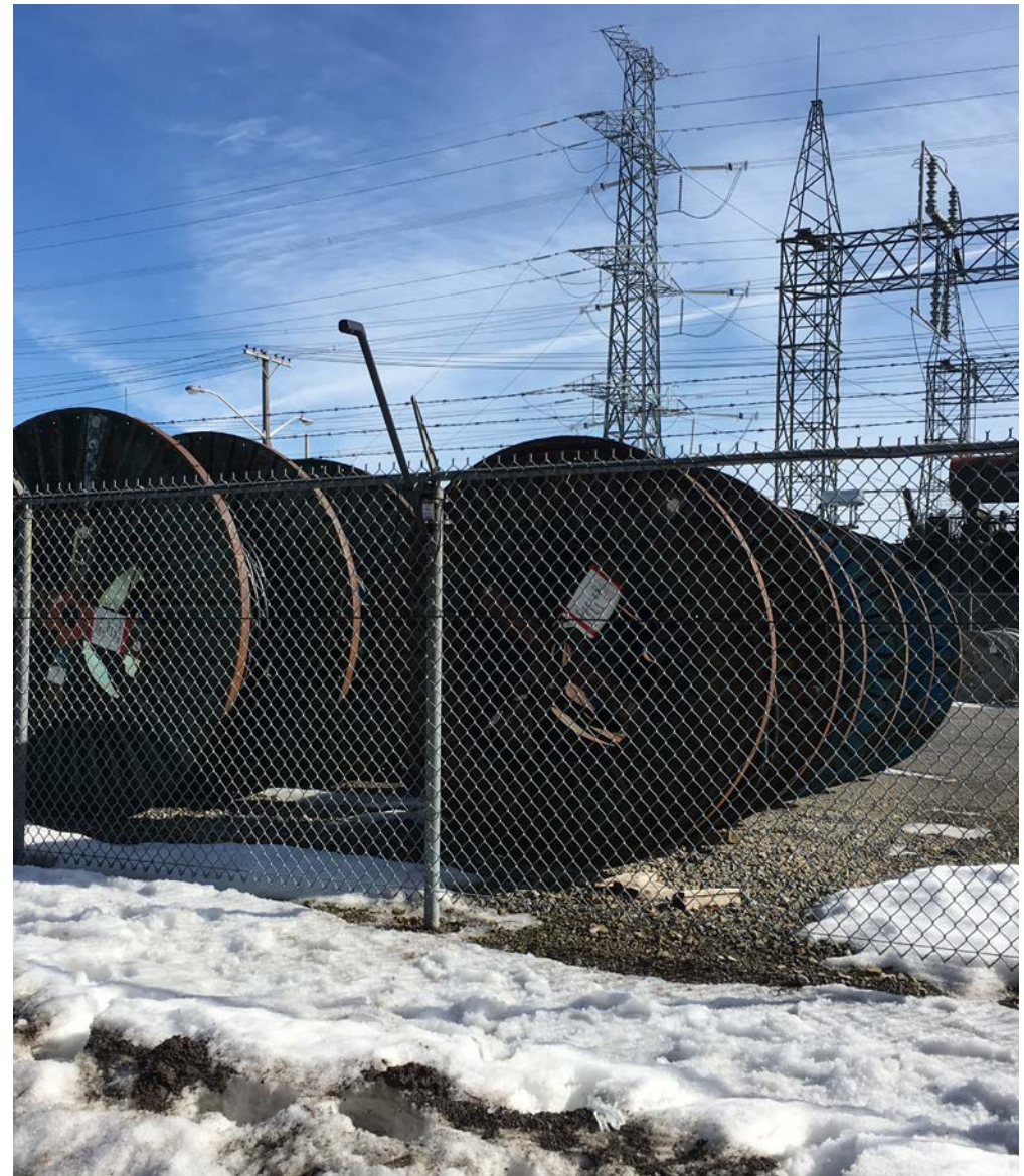
Senstar LM100 Hybrid Perimeter Intrusion Detection and Intelligent Lighting System protecting an electrical storage yard.
