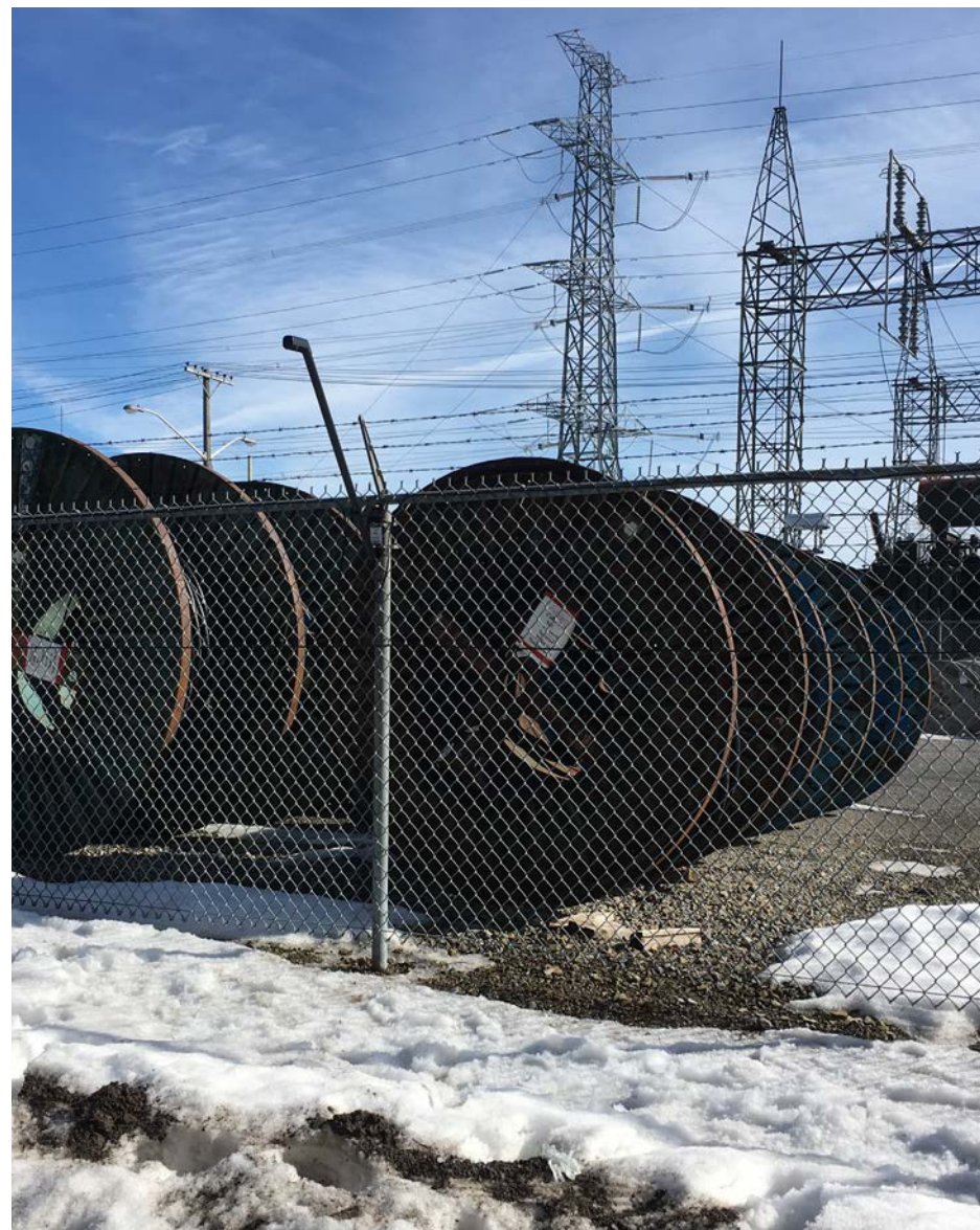
Senstar LM100 Hybrid Perimeter Intrusion Detection and Intelligent Lighting System protecting an electrical storage yard.
