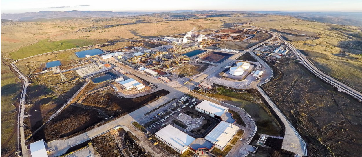
Meta Nikel Kobalt Mine Facility in Turkey
